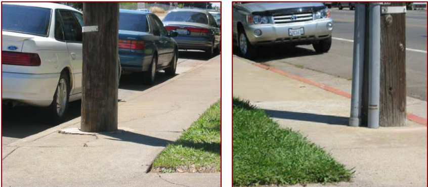
Figure 3: Utility Pole Obstruction Examples - Mather Field Road at the Mather Sports Complex and Senior Center
