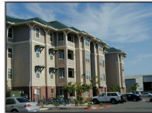
This multi-family project in Davis, California includes detailing at all levels of the building (i.e. window accents, roof overhangs) and is an excellent illustration of the base, middle, cap concept, with the base being brick, the middle being stucco, and the cap being siding.
