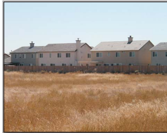
Don't Do This: This single family project does not have any variation in roof planes.
