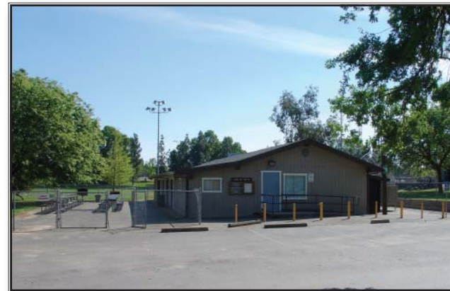
Don't Do This: Community building at a park with minimal landscaping; unidentified pedestrian access; and unwelcoming seating area. (Fair Oaks, California)
