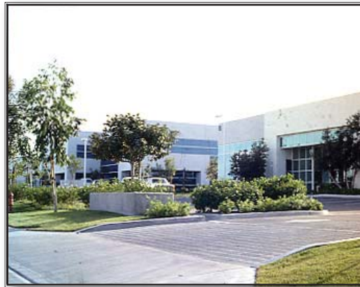
Site access to this industrial project is designed to allow easy circulation throughout the site. (Courtesy LPA)
