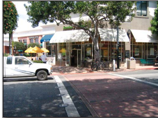
Example of a mid-block crossing in San Luis Obispo, California. The crossing features special paving, paint striping, a bulging of the sidewalk to narrow the street, and special lighting in the street that flashes when pedestrians are in the crossing.
