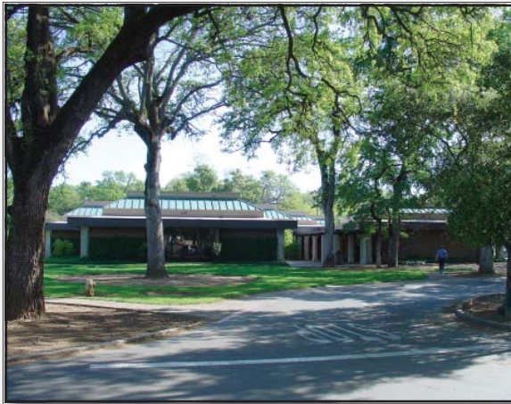
Do This: Library facility built within existing grove of trees (Sacramento County, California).
