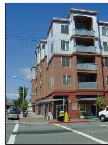
This residential mixed-use project in Oakland, California illustrates the concept of base-middle-top. Each segment of the building (ground floor, middle, top floor) is characterized by a change in materials, color, or architectural detailing, breaking up the building mass vertically. Additionally, the varying roof lines and projections/recesses of the façade break up the building horizontally.
