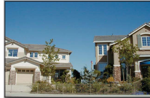
This multi-family project includes articulation of the wall, trim around the doors and windows, and accents at the entries to the units to break up the mass of the structure.
