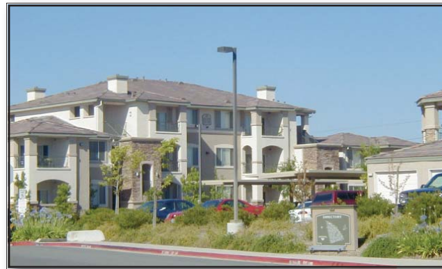
This multi-family development in Roseville, California places the taller parts of the buildings at the center and tapers the height down towards the outer edges. This helps to reduce the mass and scale of the building.
