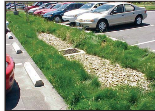
A bioswale around a drain inlet. The design allows for rainwater and irrigation runoff to be filtered before entering the storm drain system, helping to keep area rivers and creeks clean and safe.
