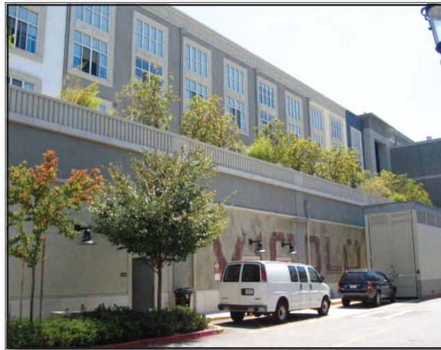
The service area at Santana Row, San Jose, California. Landscaping is used to soften the built form. The walls of the building include design features and murals that make the surface pleasing to look at. Large trash receptacles are contained within a fully enclosed structure to hide them from public view.
