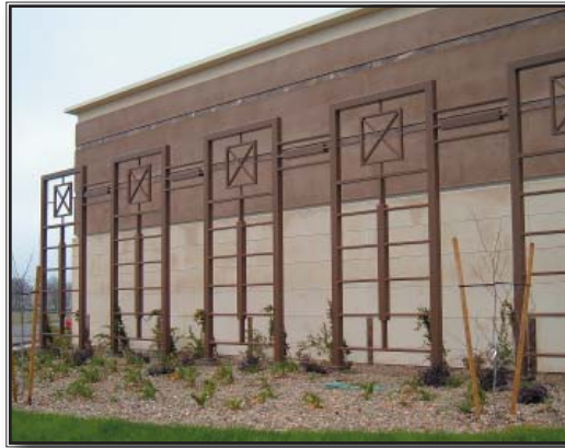
This medical building utilizes a trellis structure to add visual interest to the building elevation.
