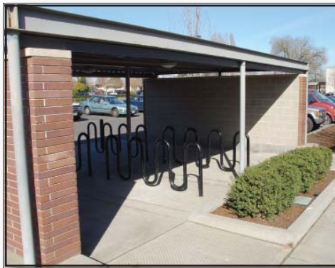
A designated bicycle parking area in a highly visible location (Beaverton, OR).
