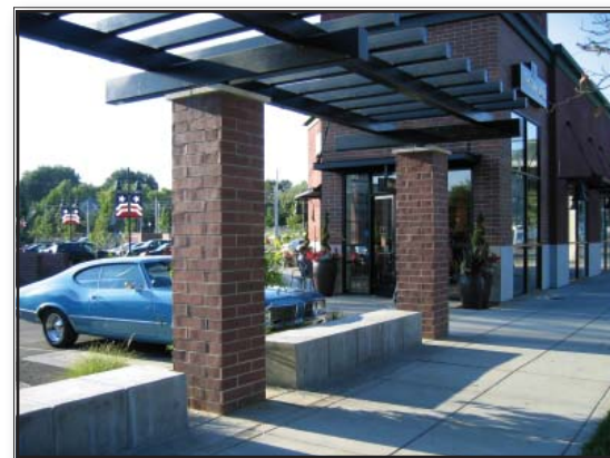
This pad building at 19th and S Streets in Sacramento is located close to the street and includes pedestrian amenities (the trellis work) that connect it to the sidewalk. The trellis includes seating areas for pedestrians and appropriate landscaping to soften the appearance of the site.
