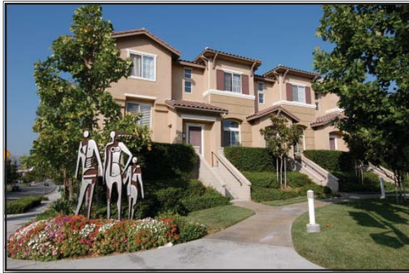
The massing between these two homes in Folsom, California is complementary. The second floors are set back farther from the street than the first. Horizontal elements, including the trim and wainscoting, break up the structures vertically. Neither home dominates the other.
