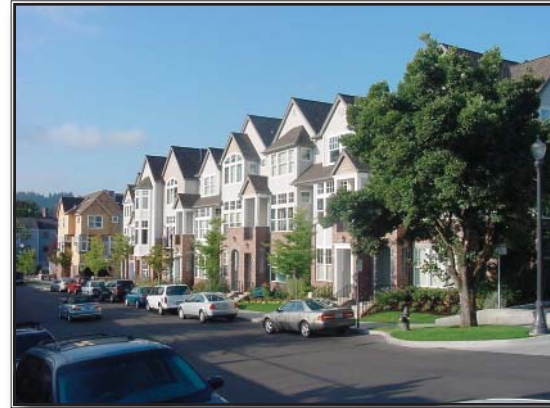
Residential development in Lake Oswego, Oregon. The façade of the buildings is rich in detailing, with brick along the first floor of the building and trim around all the windows. The walls are articulated often to break up the building horizontally.
