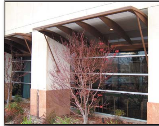
Awning are used to add interest to the façade of this industrial building.
