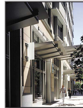
Protection from the elements is provided through the use of overhangs and awnings like these.
