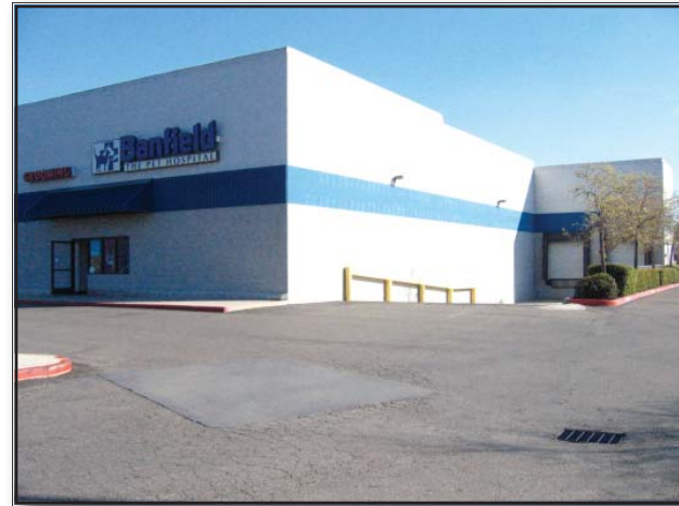
Don't Do This: Commercial Project in Rancho Cordova, California. The loading area is on the side of the building and is completely visible from the street.
