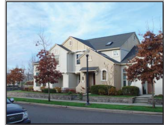
This picture illustrates a triplex, which has been designed to fit into a neighborhood with single family homes. The three units share a parcel, but each unit is individually owned (land owned in common). (Orenco Station, Portland, Oregon)
