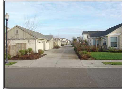
This single family development in Orenco Station, Hillsboro, Oregon uses a rear alley concept where the garages are located.
