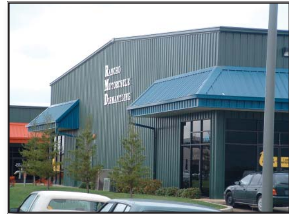
The signage at the Rancho Motorcycle Dismantling in Rancho Cordova, California is integrated with the building style and scale and does not visually detract from the site.
