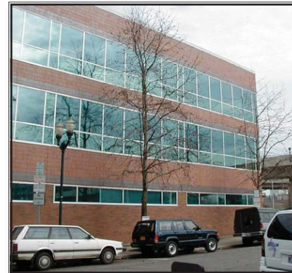
Don't Do This: Window style and flat surface provide little visual interest to this façade. High windows on the ground floor are not inviting to the pedestrian (Portland, Oregon)
