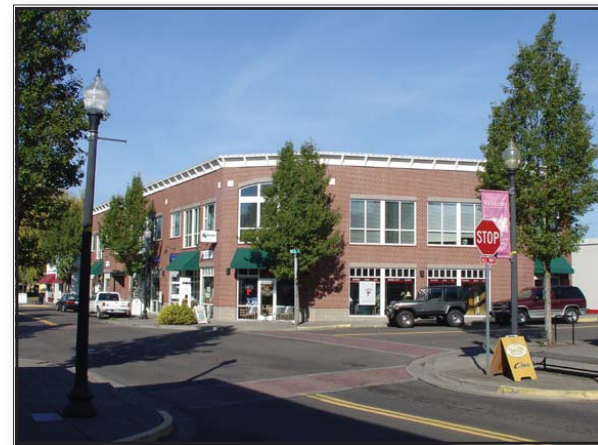
A commercial-office development in Gresham, Oregon. It is built close to the street with store fronts that are attractive and inviting.
