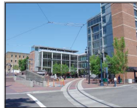
The Light Rail line runs through the middle of this project. The station is integrated into the overall design and character of the site. (Urban Studies, Portland, Oregon)
