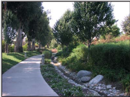
Do This: Walking/bike trail that includes natural landscaping and drainage features. (Courtesy LPA)
