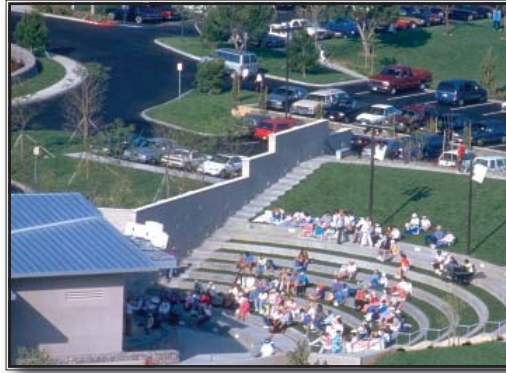
This sports complex provides for a variety of facilities for sports and other group activities, such as an outdoor amphitheater (Temecula, California, Courtesy LPA).
