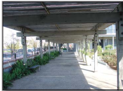
Covered pathway adjacent to public open space area. (Citrus Heights, California)
