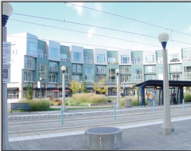
Do This: This residential mixed use project in Beaverton, Oregon is integrated with the light rail stop, promoting a high level of connectivity between the uses and encouraging transit ridership. The station is lighted and landscaped to create a pleasing, safe environment.
