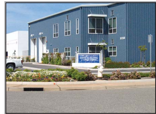
Light industrial project in Rancho Cordova, California.
