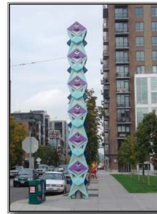
Art can be used to screen or enhance structures, such as this totem pole in the Pearl District of Portland, Oregon. It is covering a pole that supports the overhead power lines for the streetcar line.
