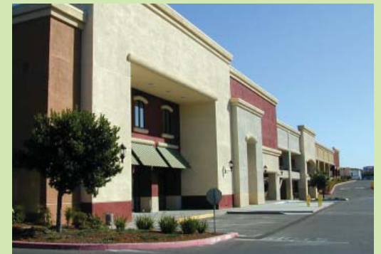
Service area concealed in architecture adjacent to building entry
