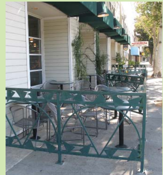
Building articulation along the public sidewalk creates extra depth to allow for outdoor dining and adds visual relief.
