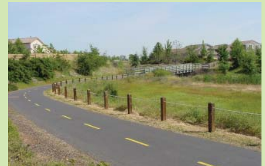
Class I trail with post and cable fencing defining the trail edge
