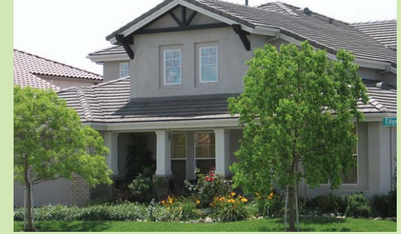
Architectural detailing and articulated facades lend interest to building form.
