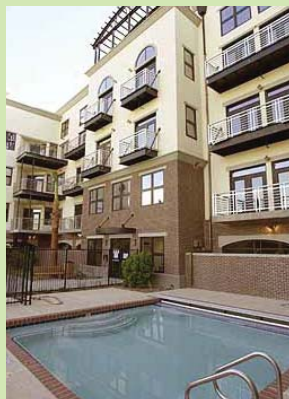
Courtyard view of podium unit © DESIGNLENS
