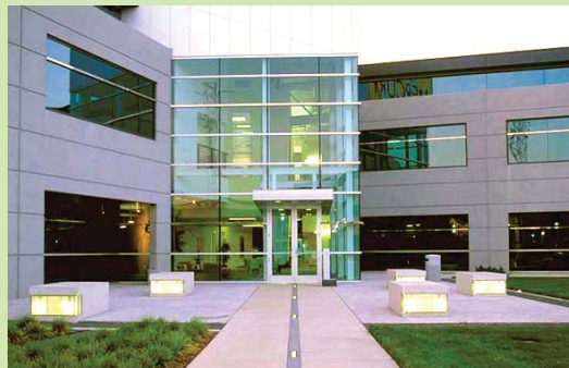
Modern architectural styling with glass and steel at the building entry helps to break down the mass of the concrete panels.
