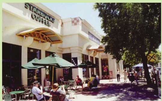
Inviting retail street has parking to the side and rear of the building.
