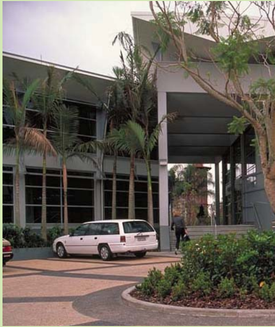
Guest parking identified by special paving at building entry
