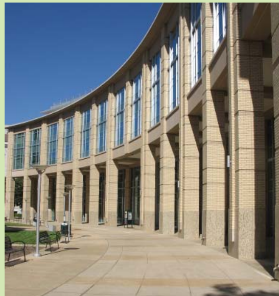
Office building architecture displaying a base, middle, and top that are appropriately scaled
