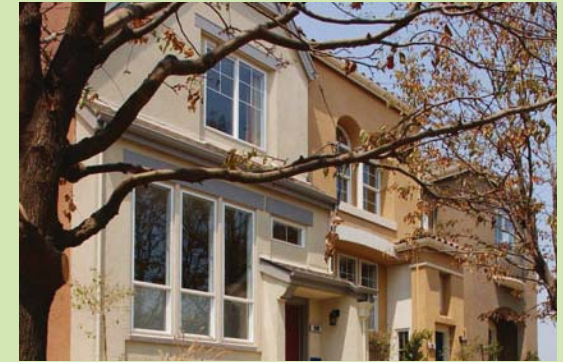
Vertical windows of varied size and shape help to minimize the appearance of mass.
