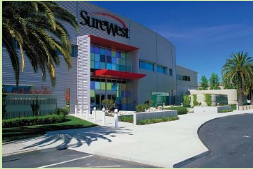
The formal entry of this industrial building relates well to the street.
