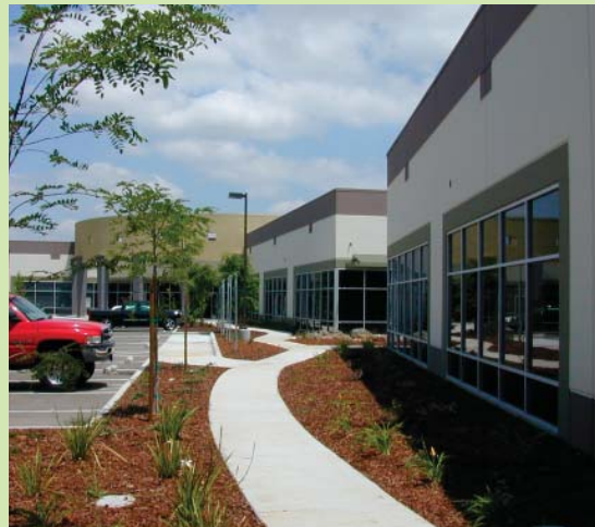
Multiple-tenant industrial complex anchored by common lobby area
