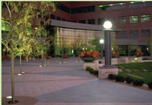
Uniform lower level lighting that is distributed provides higher visual comfort than a single high-output luminaire.
