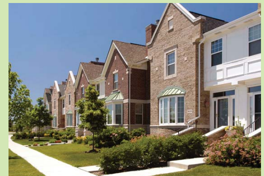
Brick or stone facades provide authenticity and richness to the building.
