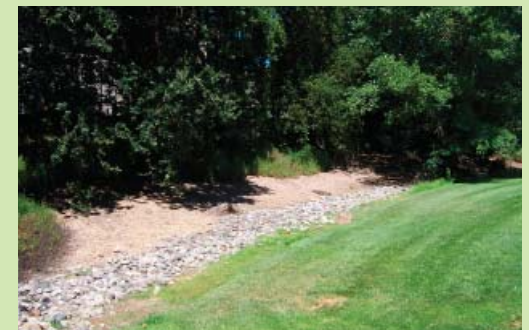
Drainage swale located at bottom of slope
