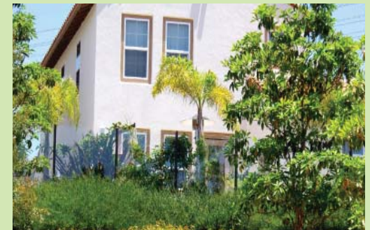
Glass soundwall used as innovative way to minimize noise while maximizing visibility
