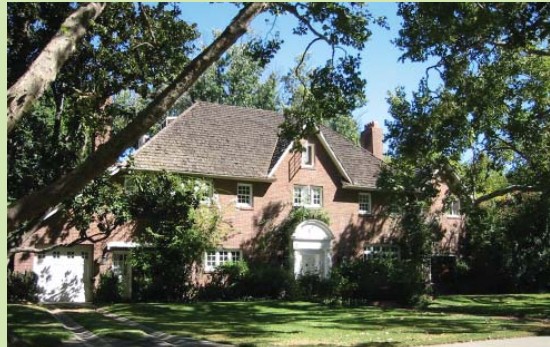
Example of an executive home single-family residence on a one-half acre lot
