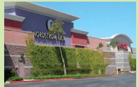
Rear of commercial buildings with screen wall
