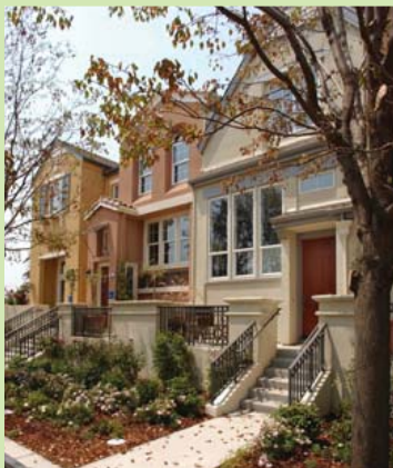
Elevated front entries with garages one-half story lower, accessed from alley © DESIGNLENS
