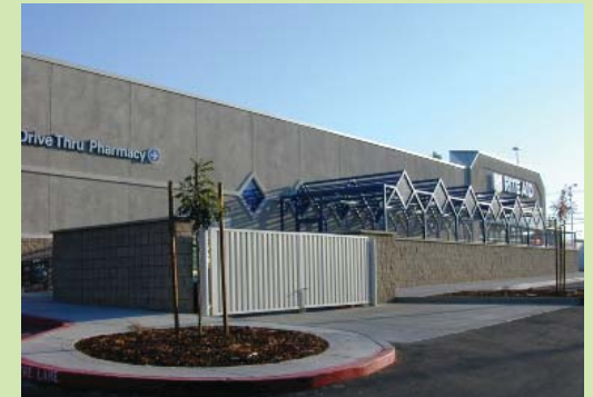
Service area hidden by architectural feature
