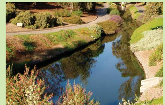
Sinuous drainage channel with varying side slopes
