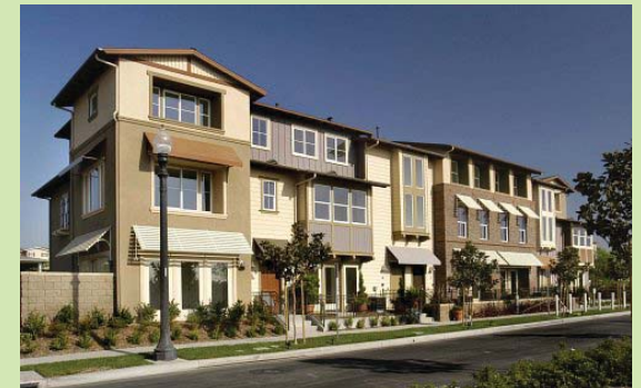
First-floor units may have direct entry from adjoining streets © DESIGNLENS
