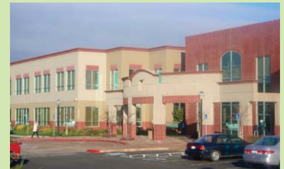
Building mass is reduced by emphasizing the building base, entry, materials and detailing.
