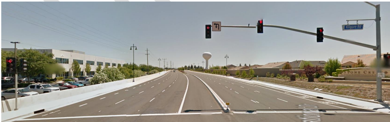
Figure 2: Looking east from Kilgore Road along International Drive. The Stone Creek residential development is largely hidden behind the long wall on the right in this image.
