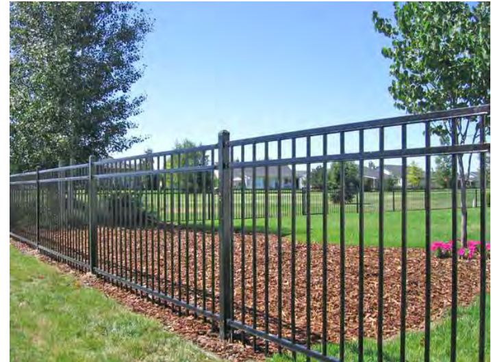
Exhibit 41: Open View Fencing
