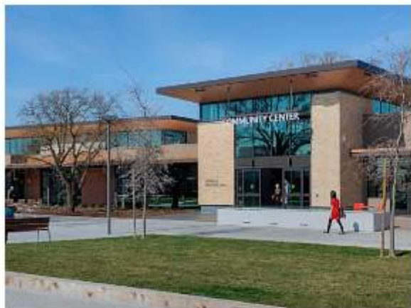
Elk Grove Community Center (Within "District56")
