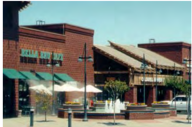
Cornice Detail and Variety of Roof Types
