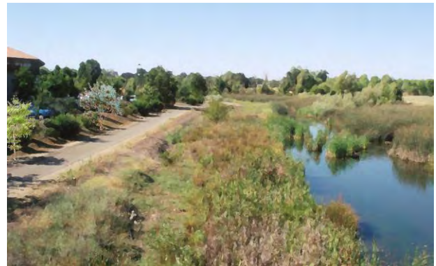
Example of naturalized drainage channel.
