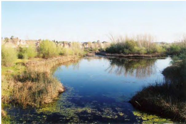
The detention basins may hold water during and immediately after each storm. However, the basins include small, permanently wet, water quality treatment ponds.
