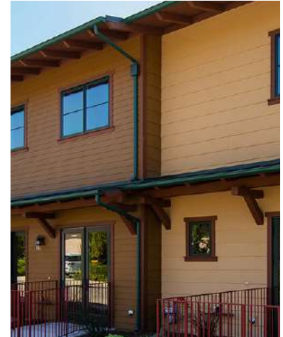
Gutter and Downspout
