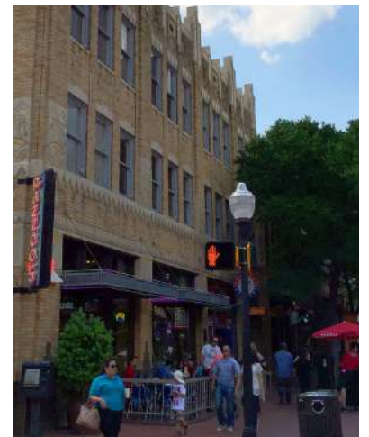
Awnings on Ground Floor
