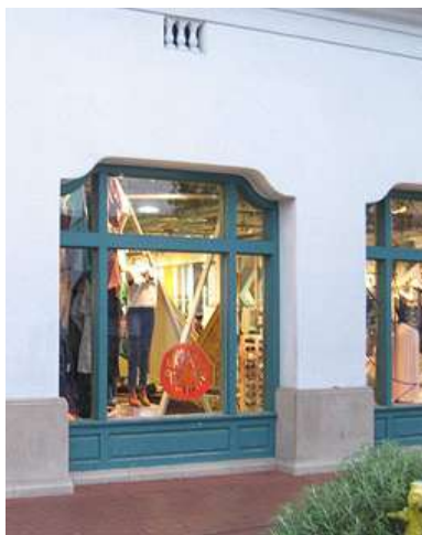
Large Ground Floor Windows
