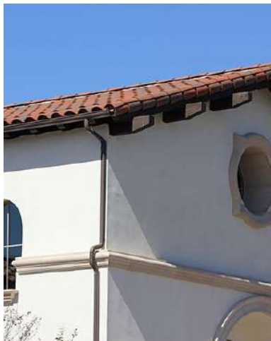
Sloped Tile Roof
