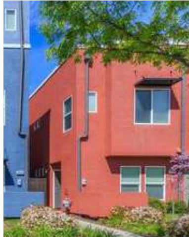
Scupper and Downspout
