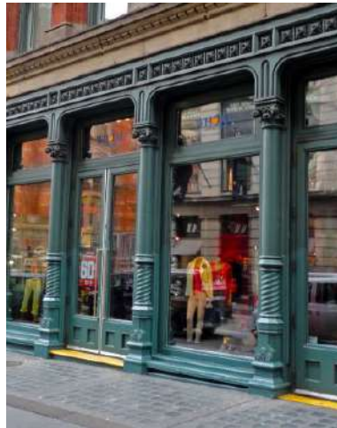
Storefront with Cast Iron Columns
