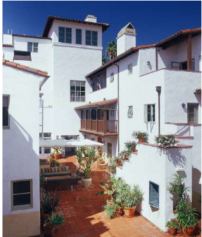
Courtyard Building Illustrative Photo Courtyard View of a Courtyard Building
