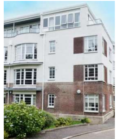
Scupper and Downspout on Side
