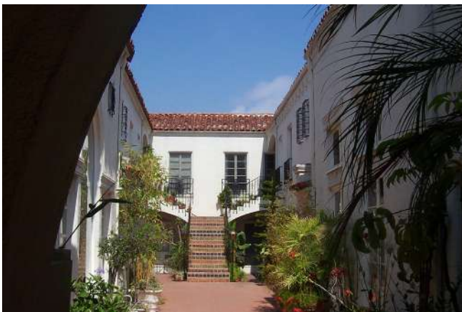
Illustrative Diagram Interior courtyards and shared open spaces should be activated with entries and windows.
