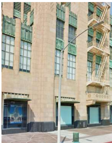
Masonry Base and Monolithic Wall
