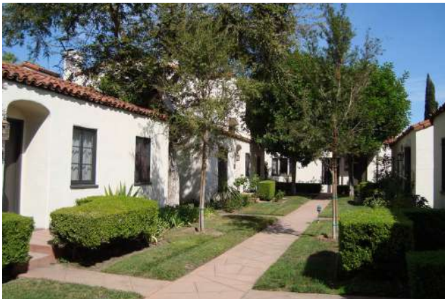
Illustrative Diagram Interior courtyards and shared open spaces should be activated with entries and windows.
