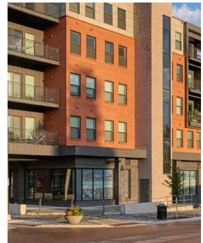
Openings Punched in Mass Wall
