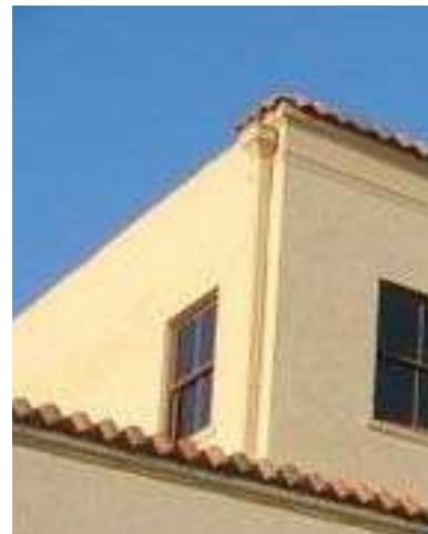
Scupper and Downspout
