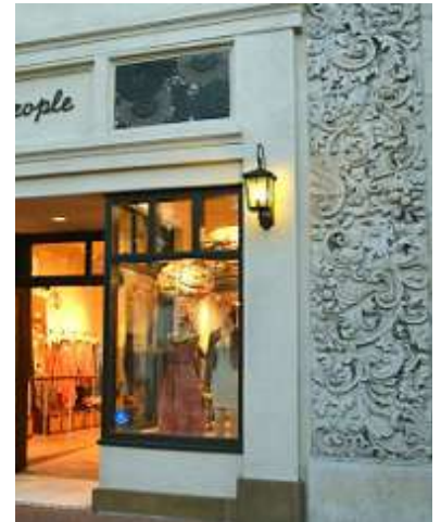
Appliqué at Cornice
