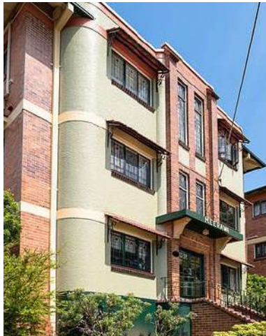
Gutter and Downspout
