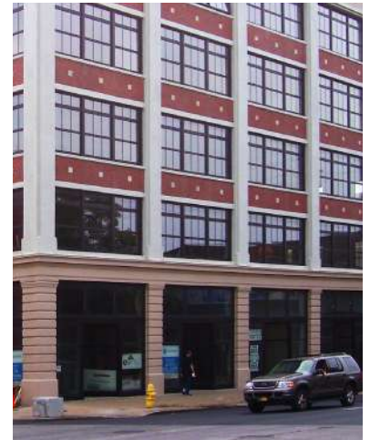
Large Windows Ground Floor
