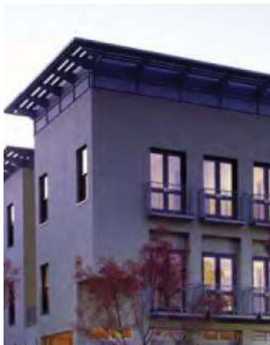
Roof Articulated with Raised Metal Overhangs
