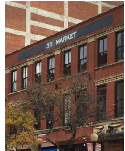
Parapet with Signage
