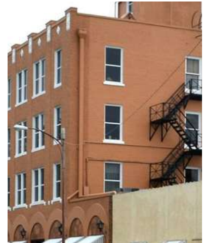
Drainage on Side of Building
