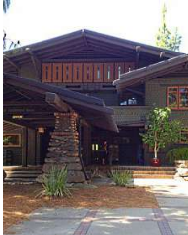
Upper Story Concealed in Roof
