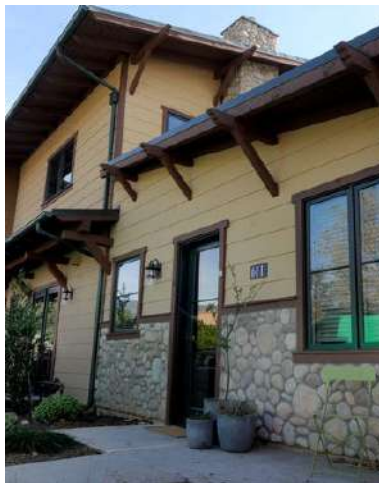
Brace and Exposed Rafters
