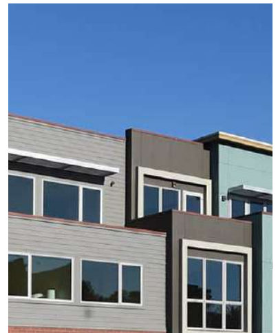
Simple Pattern Beneath Parapet with Cornice
