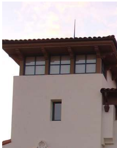
Expressed Rafters, Broad Eave
