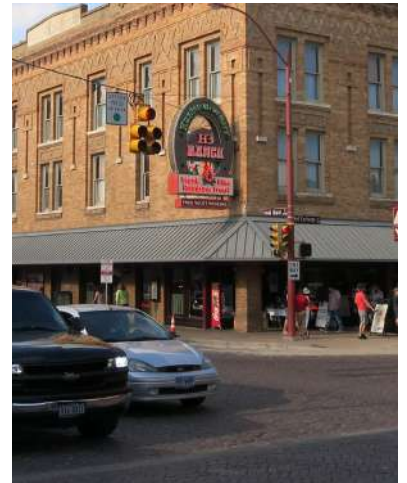
Awnings at Ground Floor Retail
