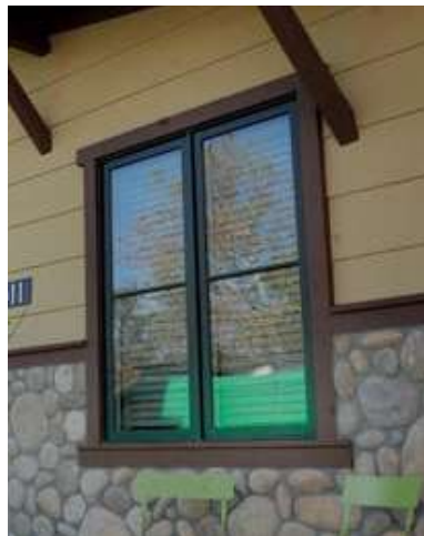
Paired Openings Composed Horizontally
