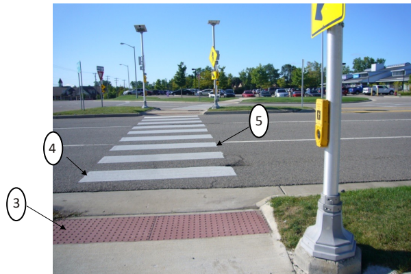
Note presence of push-button for multilane roundabout crossing. Source: Lee Rodegerdts
