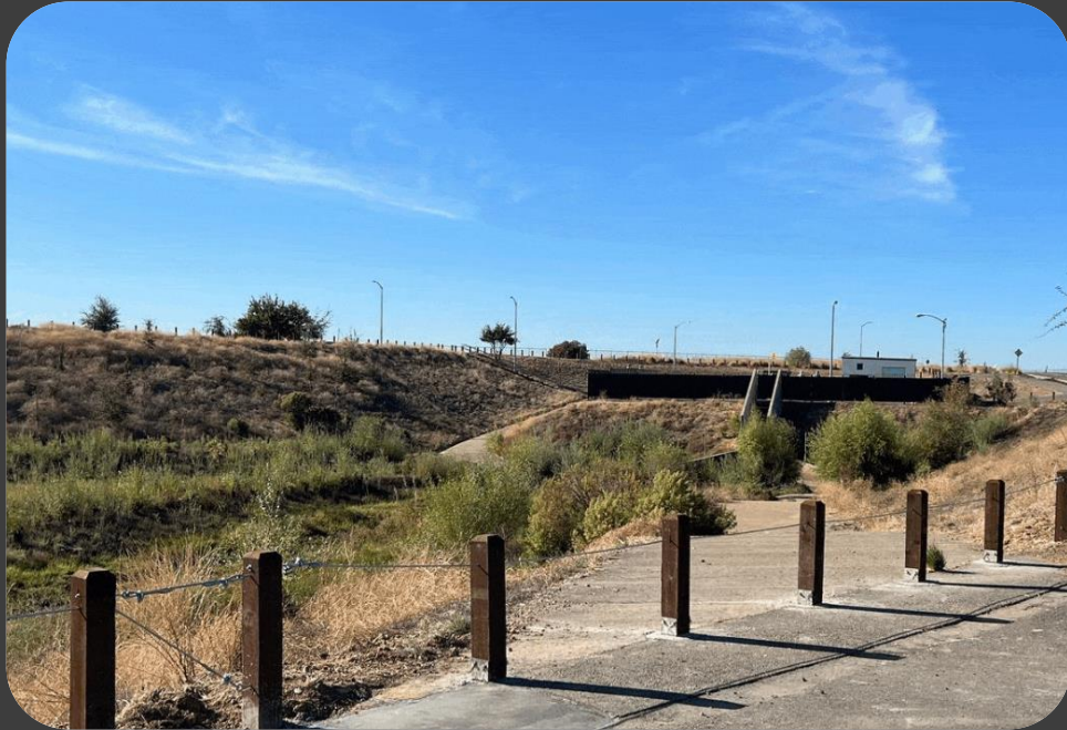
Stormwater fencing replacement program
