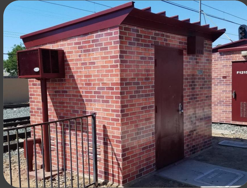
Decorative Wrap – Traffic Signal Instrument House at Folsom Blvd/Coloma Rd.
