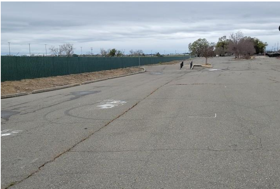
Exhibit 3.5-6 Pavement marking location for proposed signage (looking southwest)
