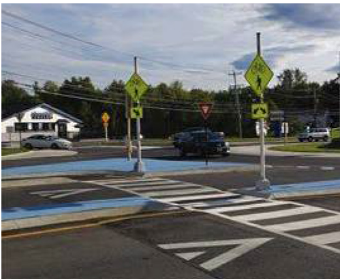
Figure F11. A Raised Crosswalk with RRFBs
