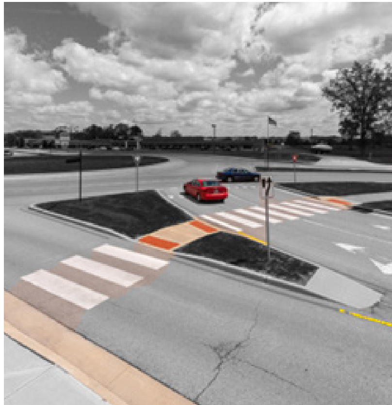
Figure F10. Two-Stage Crossing Example
