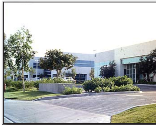
Site access to this industrial project is designed to allow easy circulation throughout the site. (Courtesy LPA)
