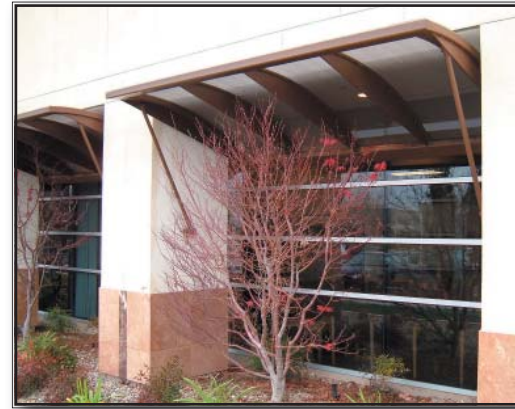
Awning are used to add interest to the façade of this industrial building.
