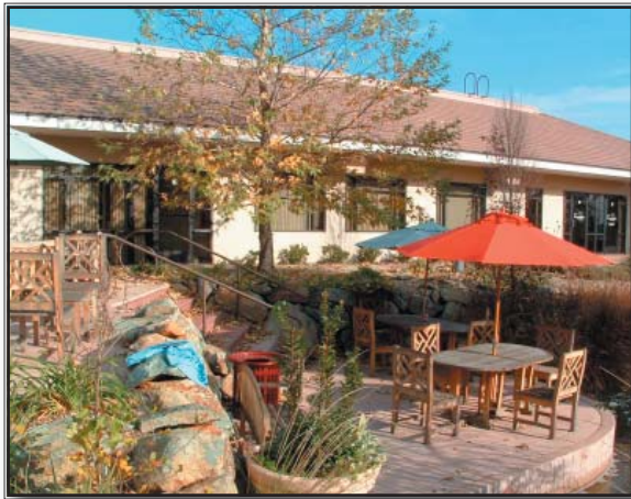
Do This: The restaurant/break area with seating, landscaping, shade canopies, and water feature is inviting and encourages active participation of the site by users. (El Dorado Hills, California)
