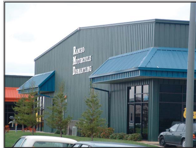
A light industrial building located in Rancho Cordova, California.
