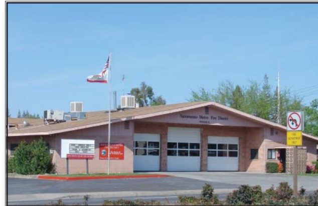
Don't Do This: Public entry to this fire station is difficult to find. (Sacramento, California)
