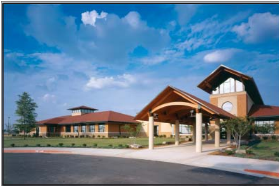
Entry with significant portico extending to sidewalk. (Helena, Arizona)
