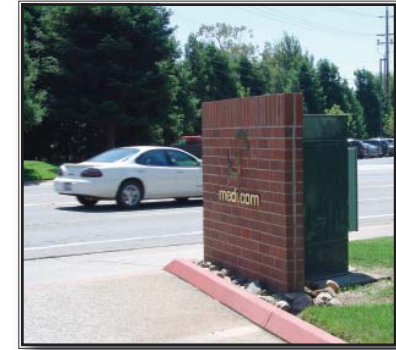
This entry sign is used to block view of metal utility box from street. (Rancho Cordova, California)
