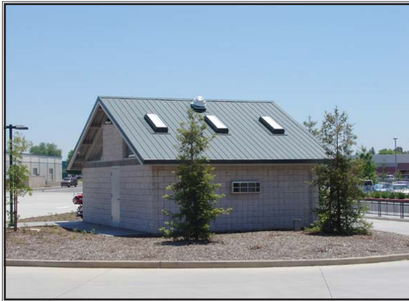
Do This: Equipment placed within a structure scaled to the neighborhood. (Rancho Cordova, California).
