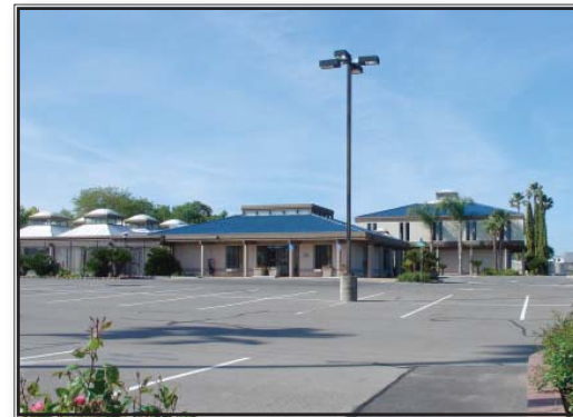
Don't Do This: Parking area lacks landscaping. (Citrus Heights, California)
