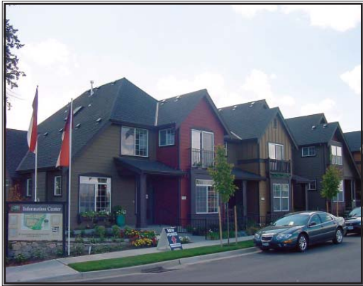
This photo illustrates single family attached dwelling units that share common walls with adjacent units. Each dwelling unit is located on an individual parcel. (Hillsboro, Oregon)
