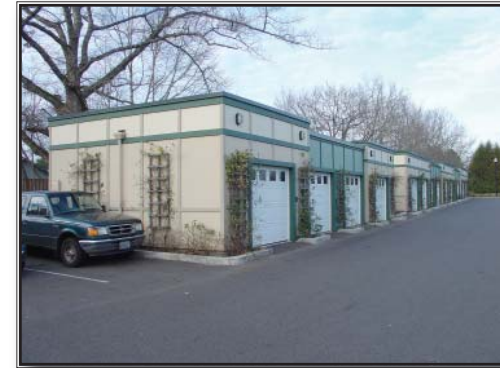
Example of garages in a multi-family project. (Orenco Station, Hillsboro, Oregon)
