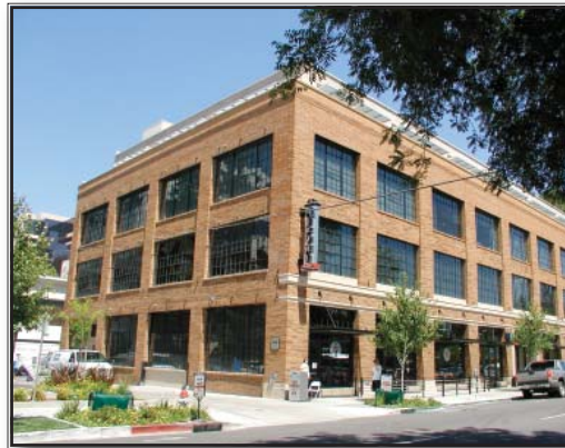
Residential lofts with retail uses at ground level (Sacramento, California).
