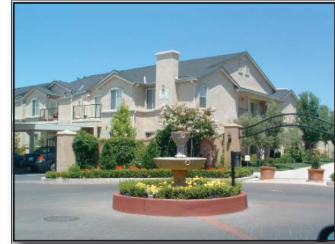
This multi-family development utilizes enhanced landscaping and special paving to alert drivers that pedestrians may be crossing.
