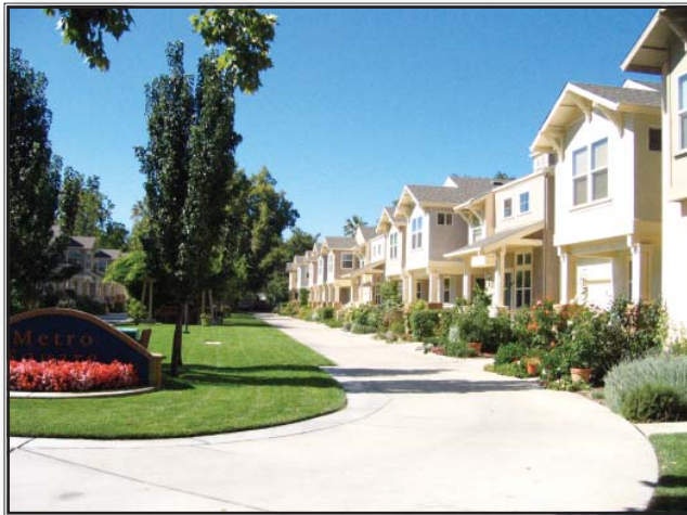
Do This: This single family project has an internal one-way loop street with individual driveways to each residence. (Metro Square, Sacramento, California)
