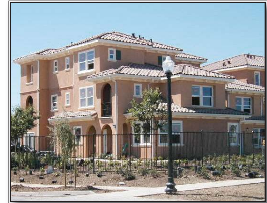
A large multi-family apartment complex in North Natomas, Sacramento, California. The scale of the project is consistent with other suburban multi-family projects, however it is variation in roof line and articulation of the façade to break up the monotony.
