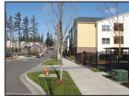
Local street provide through the middle of an apartment development with on-street parking. The parking pocket concept is used to enhance the pedestrian environment (Gresham, Oregon).
