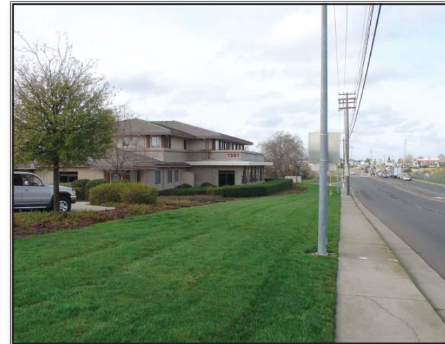
Sidewalk along right-of-way too narrow; there is no dedicated bike lane; and no pedestrian connection to the public sidewalk or the adjacent office building (Folsom, California)
