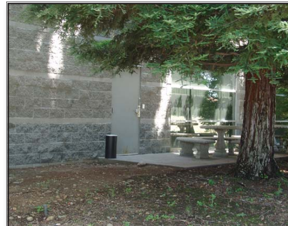
Don't Do This: Employee break area created as a design "after-thought" in a secluded remote location (Rancho Cordova, California).
