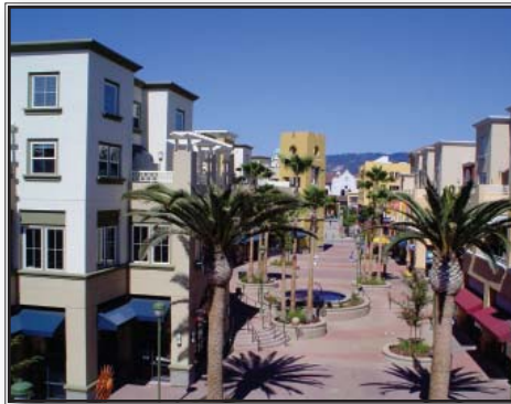
Retail and residential with pedestrian plazas and promenades at the Fruitvale BART Station in Oakland, California.
