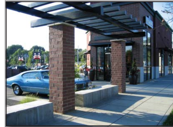
This pad building at 19th and S Streets in Sacramento is located close to the street and includes pedestrian amenities (the trellis work) that connect it to the sidewalk. The trellis includes seating areas for pedestrians and appropriate landscaping to soften the appearance of the site.
