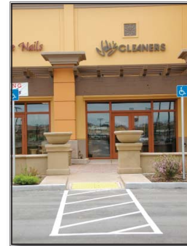
This photo shows a clearly identifiable mixing of pedestrians into the vehicular portion of the site at a development in Roseville, California. A change in color and texture are used to highlight the interaction of the two modes.
