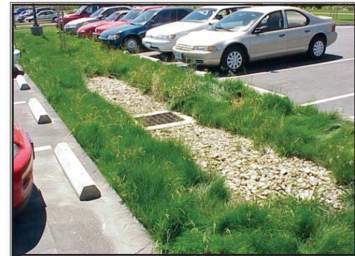
A bioswale around a drain inlet. The design allows for rainwater and irrigation runoff to be filtered before entering the storm drain system, helping to keep area rivers and creeks clean and safe.
