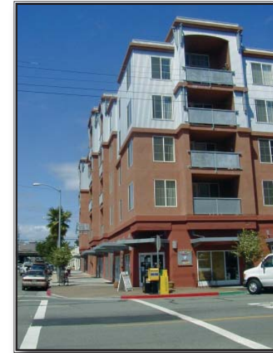
This residential mixed-use project in Oakland, California illustrates the concept of base-middle-top. Each segment of the building (ground floor, middle, top floor) is characterized by a change in materials, color, or architectural detailing, breaking up the building mass vertically. Additionally, the varying roof lines and projections/recesses of the façade break up the building horizontally.
