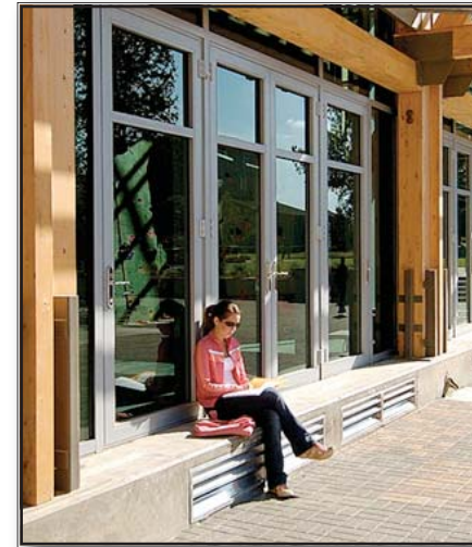
This commercial/office development includes extensive architectural detailing, such as the wood headers and trim around the windows. (Courtesy LPA)
