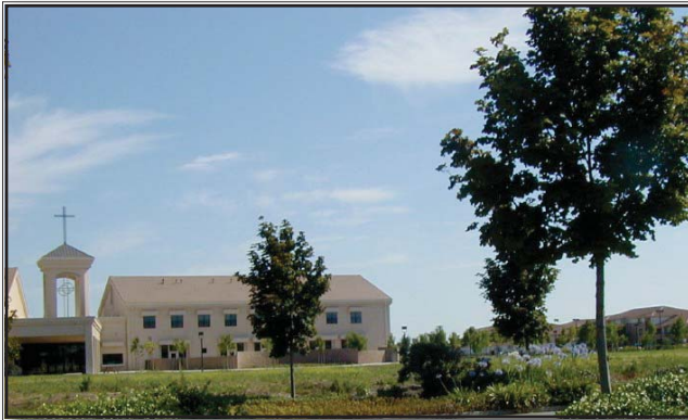
This church in Davis, California complements the surrounding residential developments by utilizing a similar mass and scale as the surrounding multi-family development.
