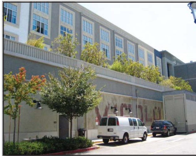
The service area at Santana Row, San Jose, California. Landscaping is used to soften the built form. The walls of the building include design features and murals that make the surface pleasing to look at. Large trash receptacles are contained within a fully enclosed structure to hide them from public view.
