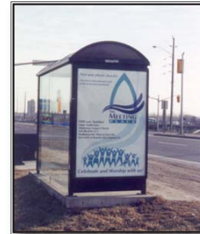
Don't Do This: Bus shelter along a suburban road. There is no sidewalk or other pedestrian connection from the stop to the street or any adjacent uses.
