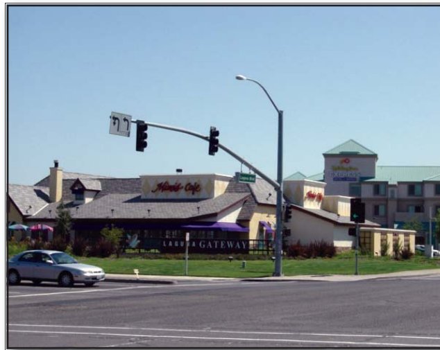
Don't Do This: Commercial center in Elk Grove, California. The site is developed with corporate architecture for its pad building that does not match with the overall style and character of the development. This does not help achieve a sense of place for the site.
